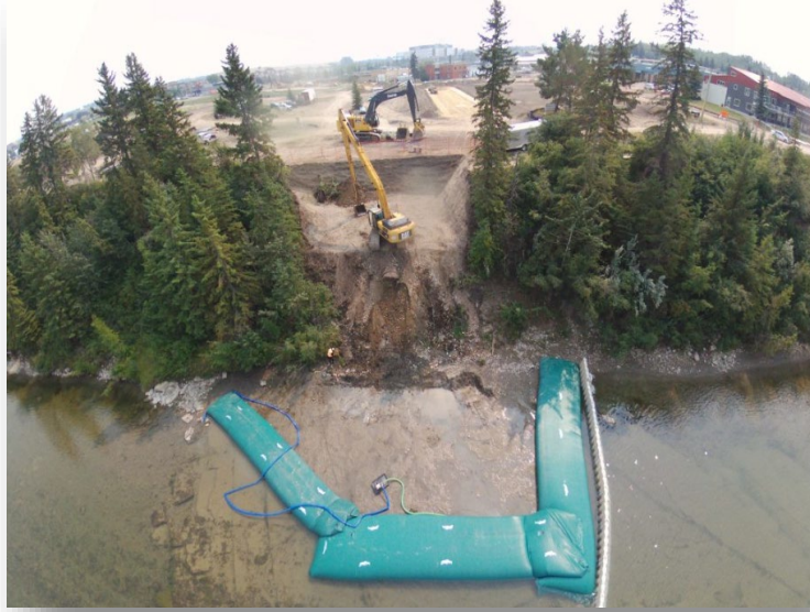
River, Stream Diversion, & Site Isolation
